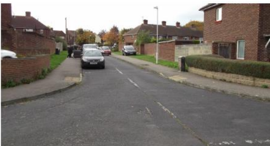
Lanes Avenue link road to Packham Road at approximately 3pm. Note the pavement and verge parking.
